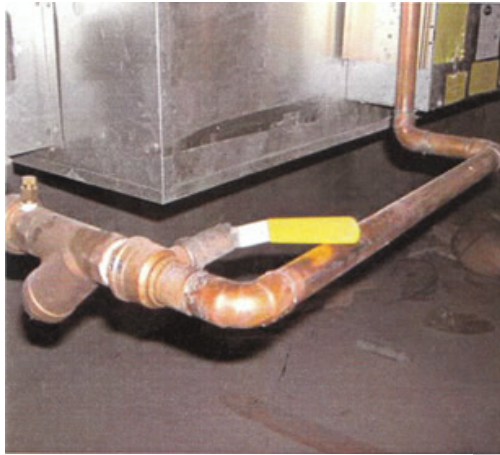
Piping design interferes with shut-off valve handle
